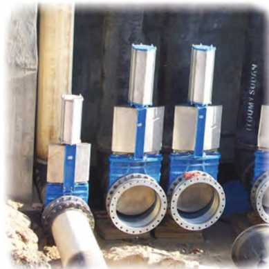
Mixing chamber installation
